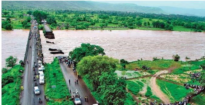
Fig. 1. Bridge collapsed at Satara on the Savitri river
