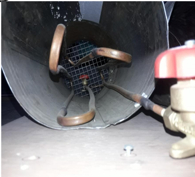
Fig-3. Condensers tubes are placed in the shell
