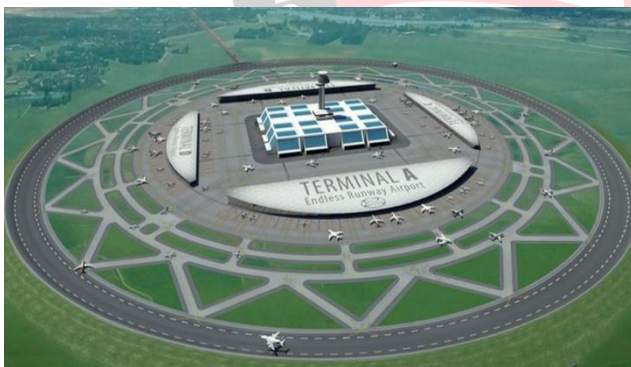
Fig. 6 Over View Of Circular Runway
