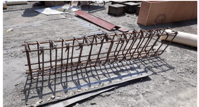
Figure 4: Type A (congested beam)
