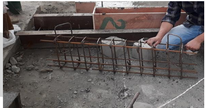
Figure 5: Type B (non-congested beam)
