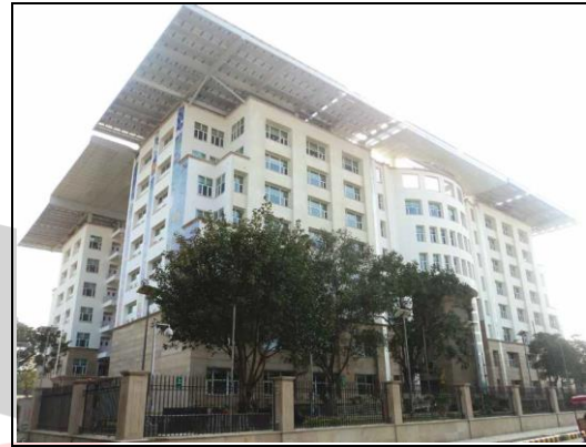
Fig. 1 North Edge Road View of The Indira Paryavaran Bhawan
