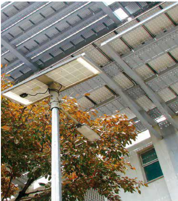
Fig. 5 Photovoltaic Power Plant at Indira Gandhi Paryavaran Bhawan
