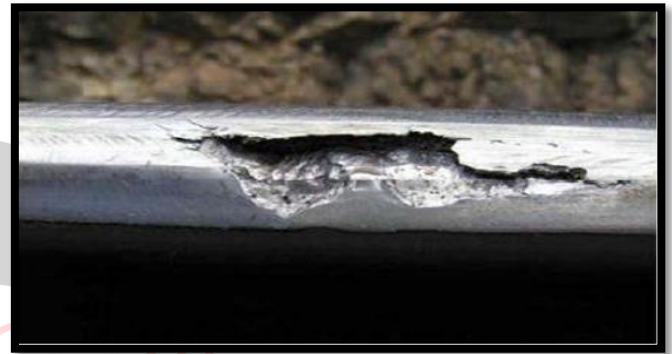
Figure 1: Typical example of broken rails (Surface Crack)
