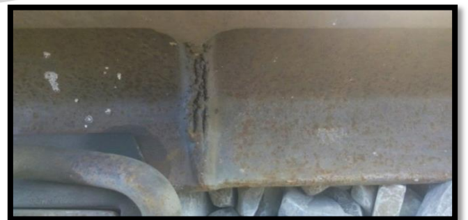
Figure 2: Typical example of broken rails (Surface Crack)
