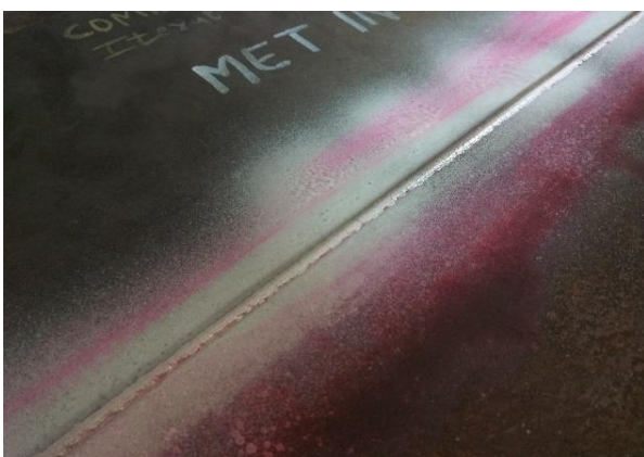
Fig. 2 DPT of the welded base plate
