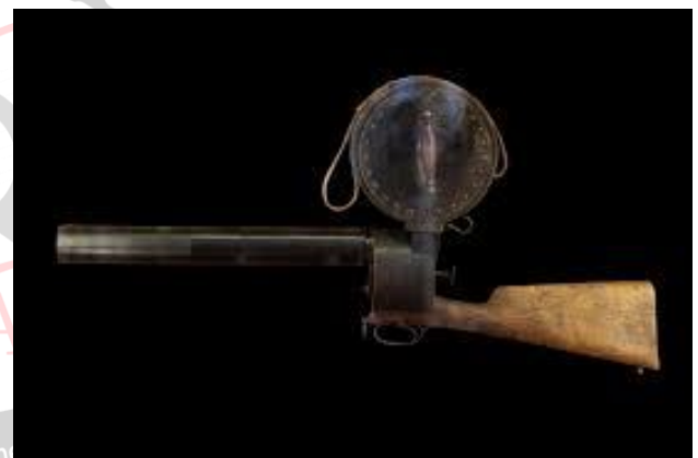
Fig. 2 Chronophotographic gun of Etienne-Jules Marey
