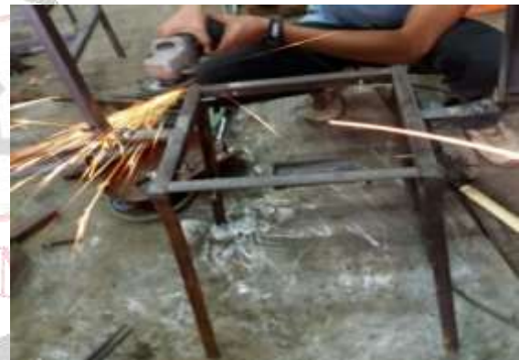
Figure 13: Grinding Operation in action
