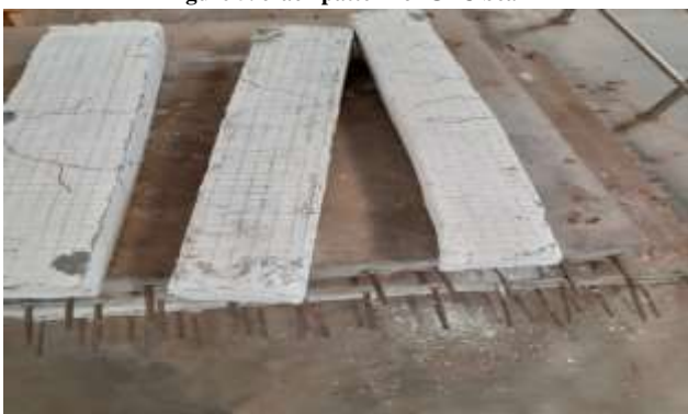
Figure 6. crack pattern of rcc beam
