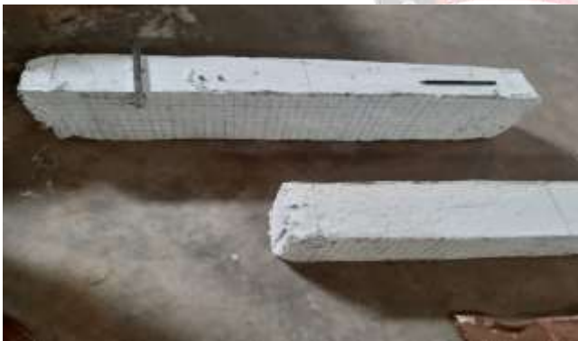
Figure 5. crack pattern of GPC beam
