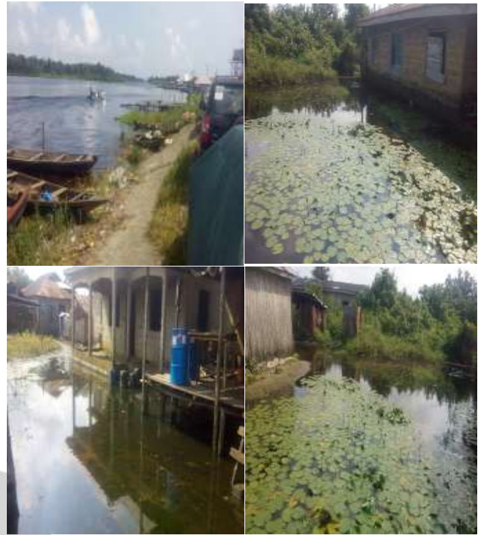
Figure 2: Diagram showing the closeness of the area to the Atlantic Ocean and how flooding is threatening the integrity of the foundation structures
