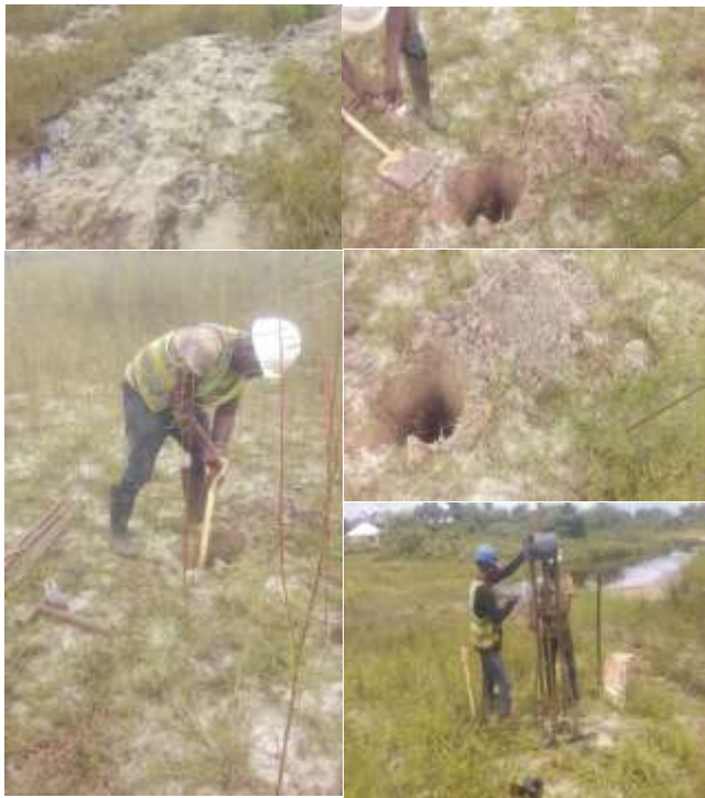
Figure 6: Field Pictures of in-situ CPT and Trial pits geotechnical tests
