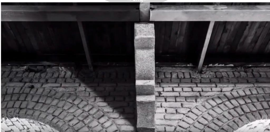
Figure 13: Stone brackets supporting the balcony above
