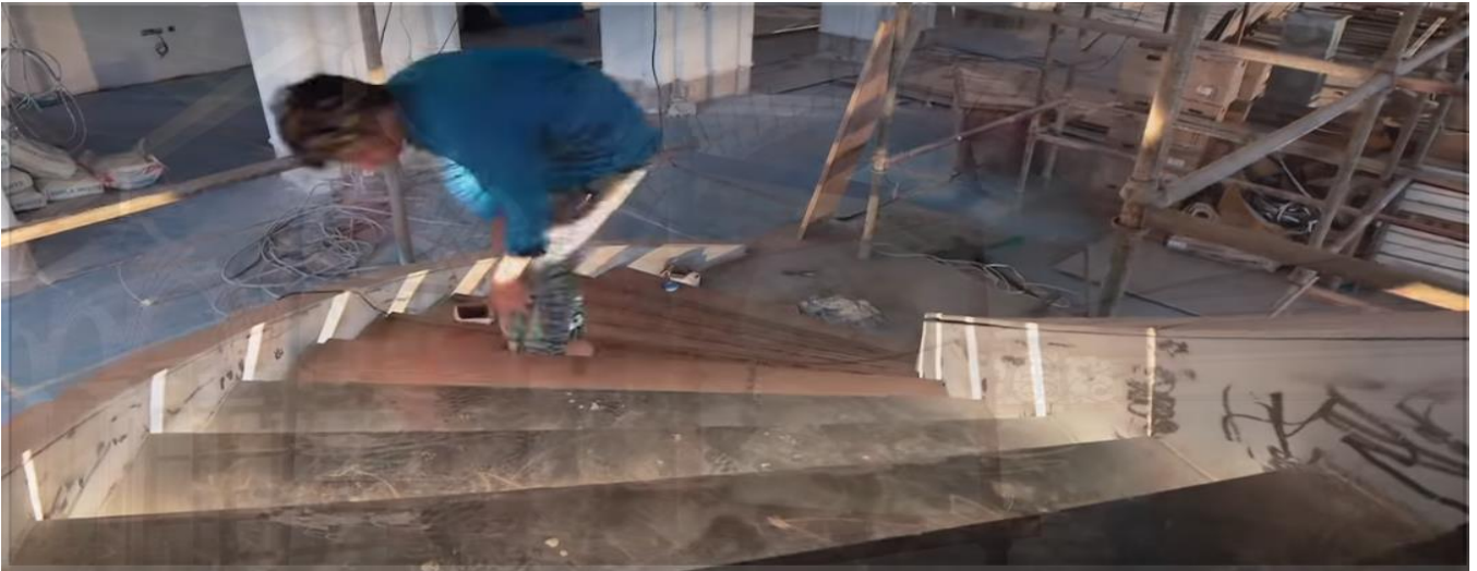
Figure 22: Construction of the new staircase inside the building
