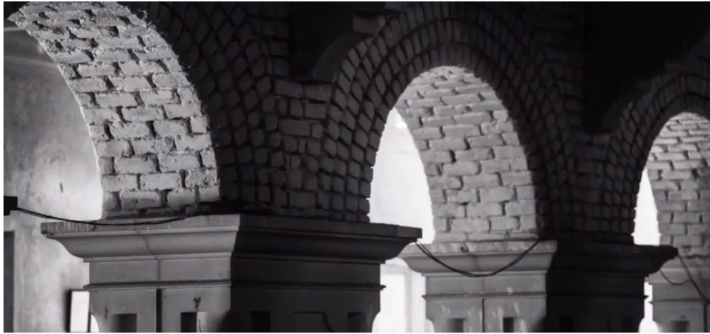
Figure 14: Semi-circular arches around the central space.
