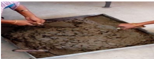
Fig: Mixing of concrete
