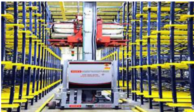
Fig.1.5 Automated Storage and Retrieval System
