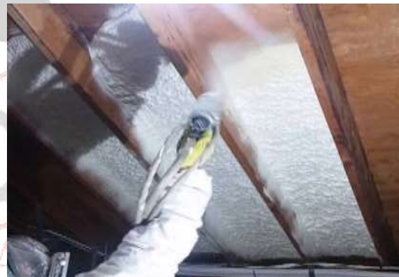
Fig 1. Showing installation of spray foam on ceiling.
