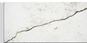
Thin Crack
