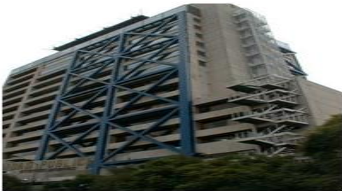
Figure.1 RC building with exterior bracing system
