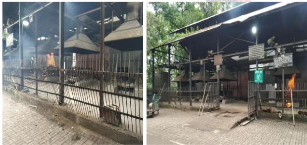
Fig No1:- Actual field photos during visit
