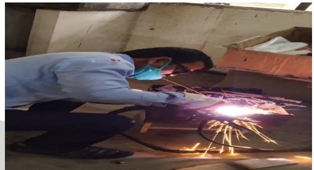
Welding the mild steel plates
