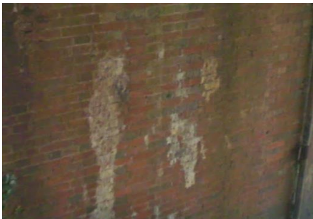
Fig. 10. Sulphate Attack Effects
