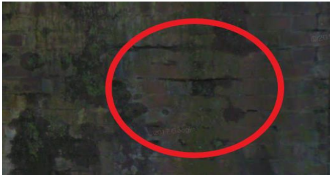
Fig. 9. Loose Brickwork
