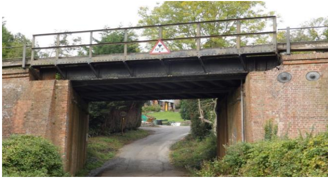
Fig. 1. The Barming Railway Bridge
