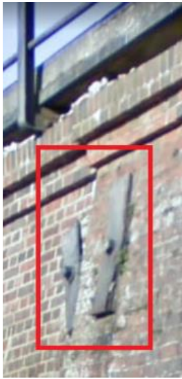
Fig. 7. Patress Plate Corrosion
