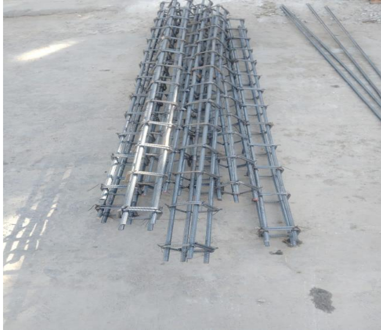
Figure 7: Mesh for Beam casting
