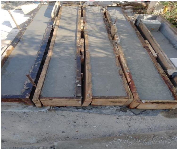
Figure 8: Wooden moulds for beam casting
