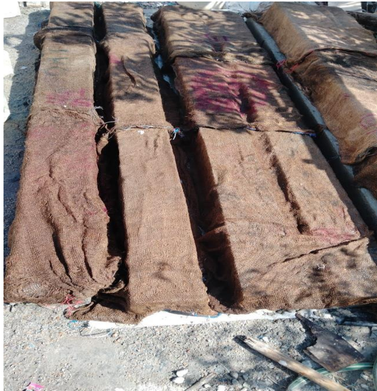
Figure 9: Curing of concrete beams
