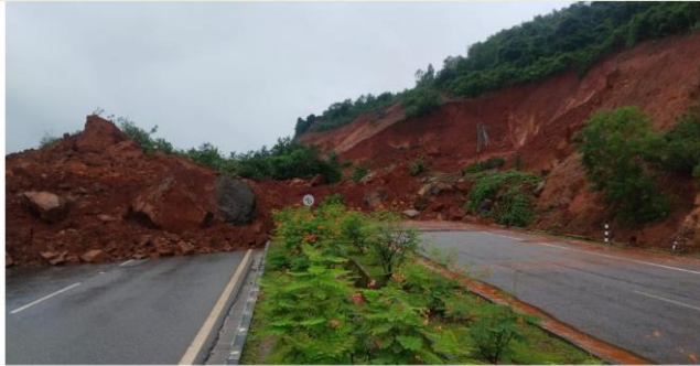
Landslide on National Highway 66 near Shirur of Ankola taluk in Uttara Kannada district on July 16, 2024. | Photo Credit: Special Arrangement
