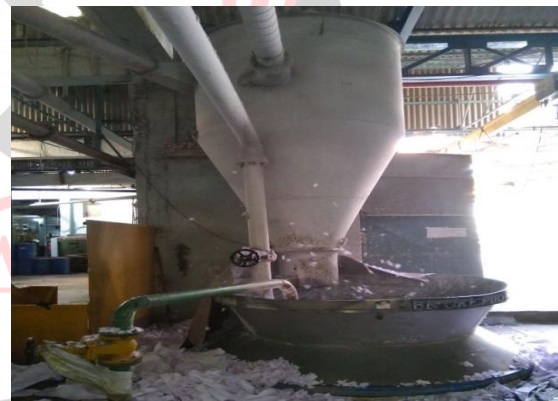
Figure 4: Cyclone connected to pulper
